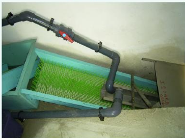
Drainage station where the fish pass has been installed
